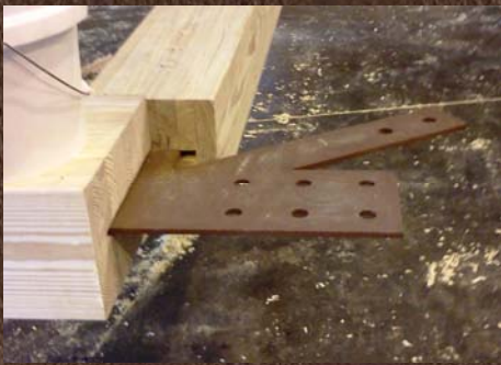
Fully concealed kerfed connections and plugged bolt holes
