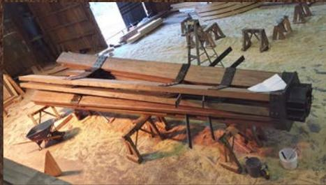
SWS partially assembled each of the "trees" to ship to the jobsite. This process not only ensures that the hardware will fit perfectly but also that the erection process will flow smoothly.
