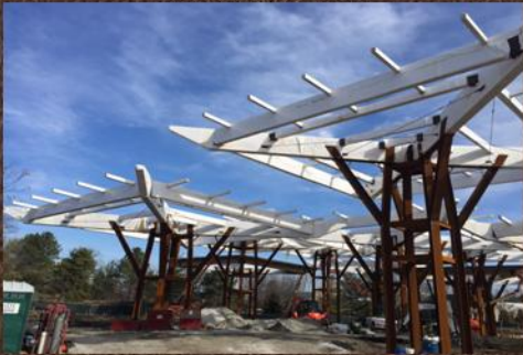
The cantilevered glulam beams are supported at the center by steel frames.
