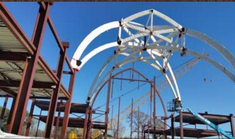
The highest peak of the glulam arches reaches 57' above the floor. This height required large cranes to lift the curved beams, pictured above, into place.
